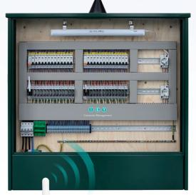
We offer a choice of three different Campère appliances. All three have the same functions and contain everything you need to wirelessly connect your guest's hook-up point with ICY Campsite Management. In addition, all three devices are equipped with a kWh meter and Ampere limiter.
